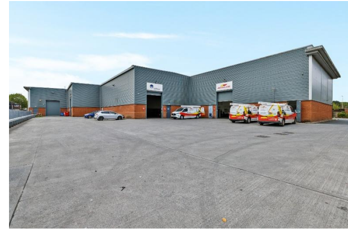
Loading Access & Yard – Units 1 & 2
